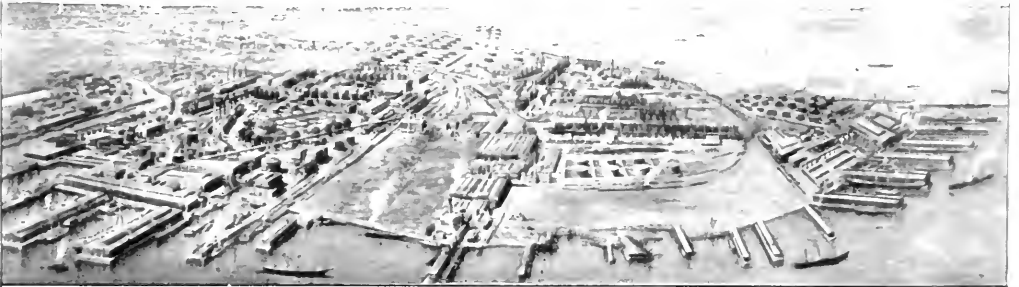
THE BAYONNE, NEW JERSEY, REFINERY
